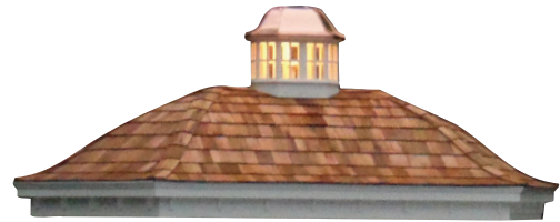
Cedar Shake Roof
